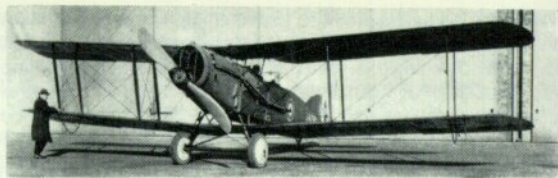
Bristol F.2B Mk. II with oleo undercarriage, enlarged tyres, flare brackets and post-war radiator shutters, 1920. This aircraft, J6790, was tested at Martlesham Heath later became G-ACCG, and survived until 1939.
