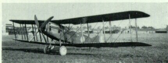
Left: Single-bay wings of 30 ft. 11½ in. span, 7 ft. chord and an aspect ratio of 4.69 were fitted first to A7860 (R.A.F. 4d engine). The Falcon-powered F.2B F4360 is here seen at the R.A.E., Farnborough, on 25th January 1923, fitted with similar wings. (Photo: Crown copyright); Right: Also photographed on 25th January 1923 was F4728, fitted with the experimental three-bay wings of aspect ratio 9.78. (Photo: Crown copyright)
